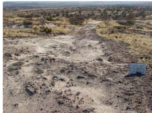
**EC-5** Erosion on route EC-A up to 12 inches.
